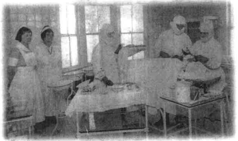
The Operating Room (c. 1920) was located in the former front parlor of the house. It was considered state-of-the-art and was lauded as the finest outside of New York City. Bright lights made surgery possible even at night.
